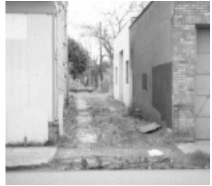
Most of the alley crossings are unpaved and lack curb ramps.
