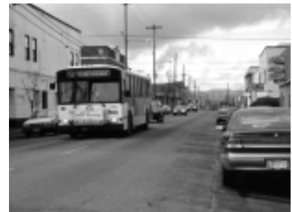
Alberta Street has one traffic lane in each direction, continuous sidewalks on both sides of the street, on-street parking in most locations, and transit service on the majority of the street.
