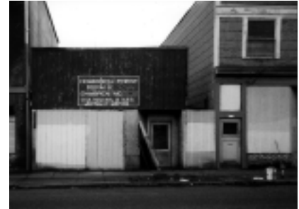
Closed businesses with boarded-up storefronts gave Alberta Street a bleak image in the 1980s.
