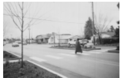
Median islands can provide refuge areas at pedestrian crossings, but also require removal of on-street parking to make room for the medians.
