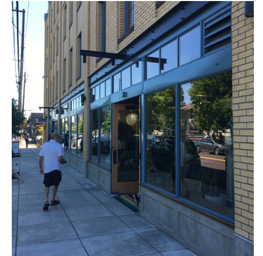
NEW BUILDING WITH NO CANOPY
