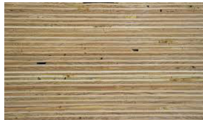
Exterior Soffit and interior ceiling - Mass Plywood
