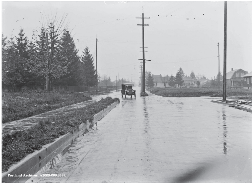
N.E. ALBERTA ST AT 31st ST LOOKING WEST, 1913
